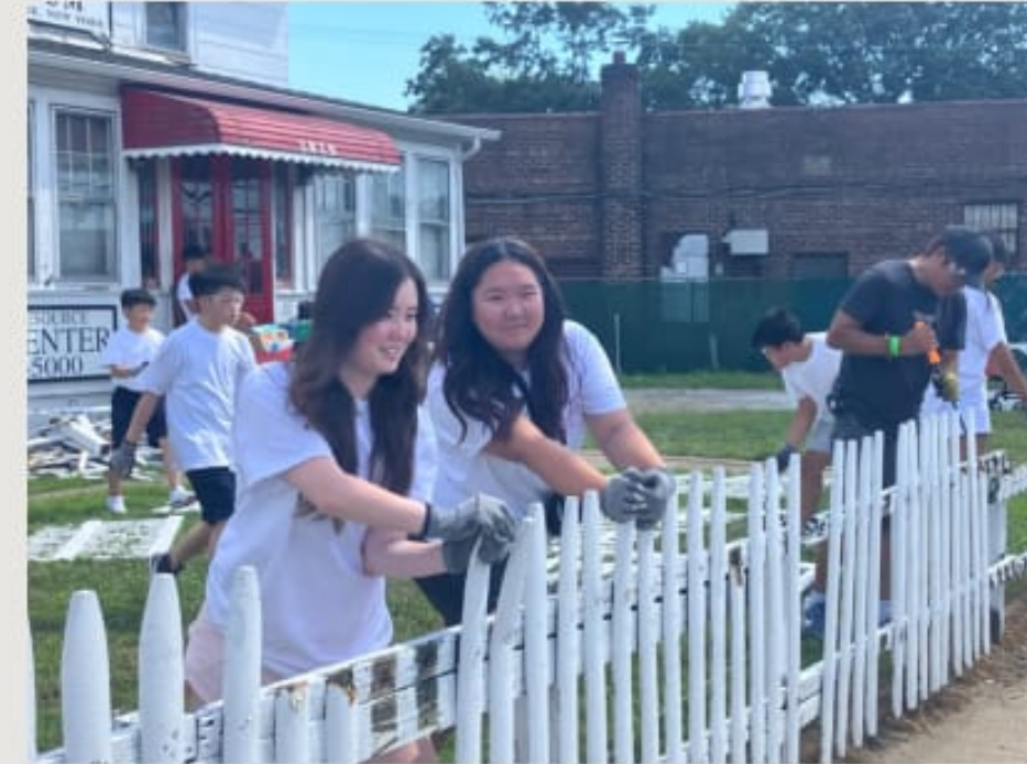
Taking down the old fence
